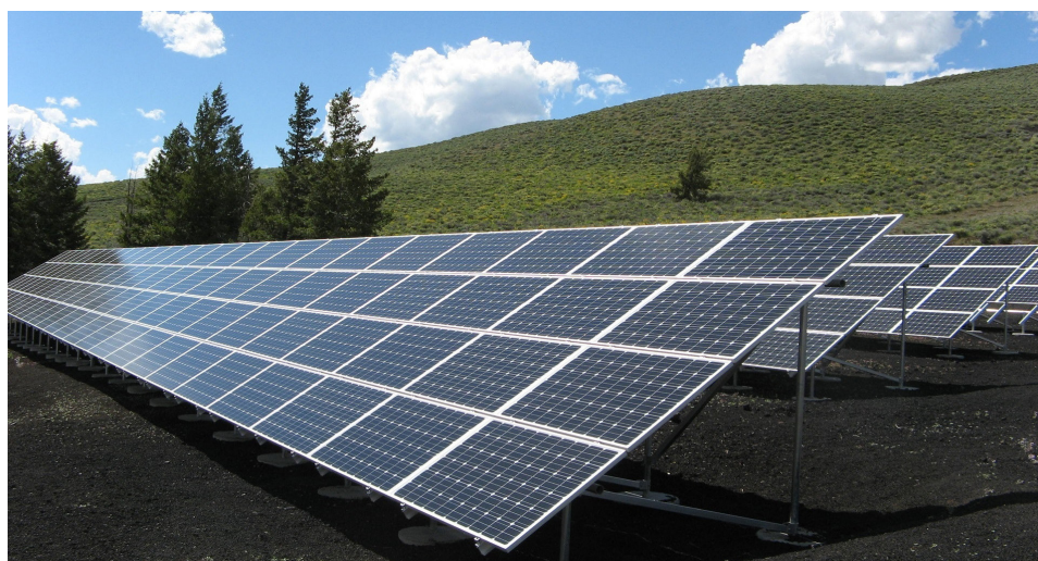
Sistem solar termic
